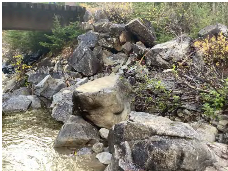
Right Bank Abutment when facing downstream
