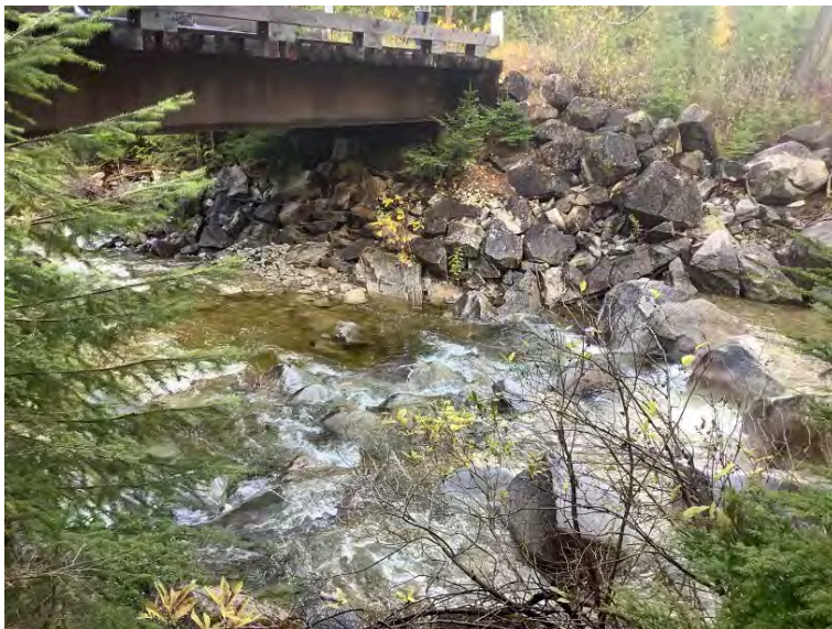
Right Bank Abutment when facing downstream
