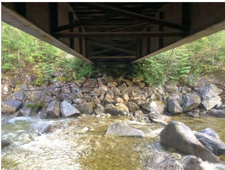
Left Bank Abutment when facing downstream
